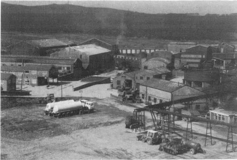
(above) Cavendish Mill near Stoney Middleton - the processing plant and offices.
